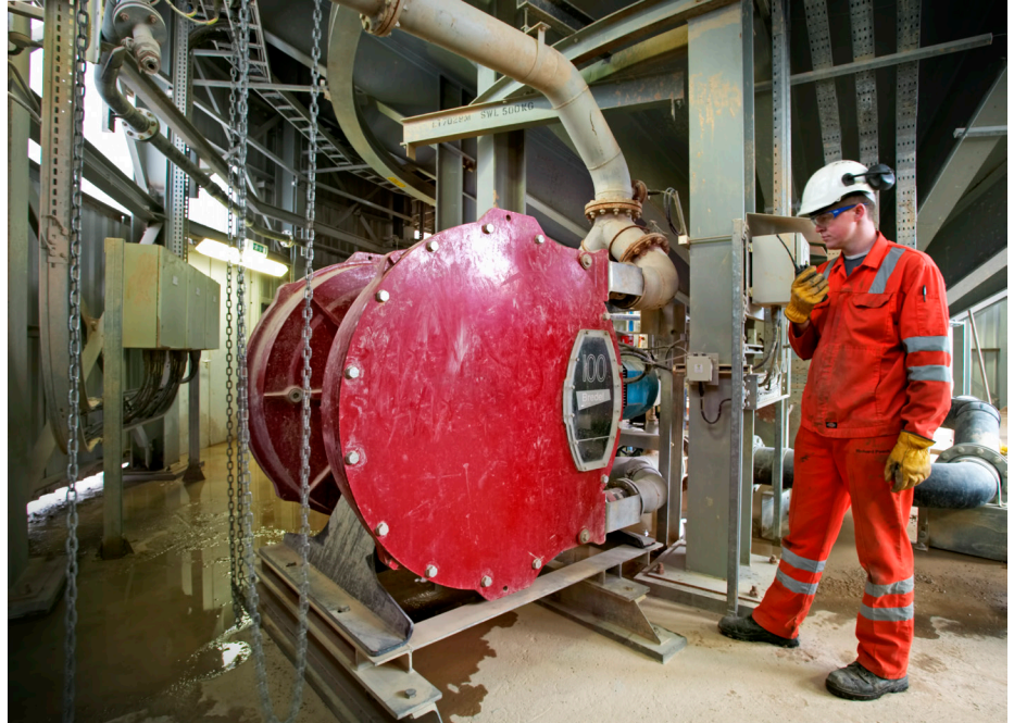
Above: Bredel hose pumps have a corrosion-resistant enclosure which suits arduous mining environments
